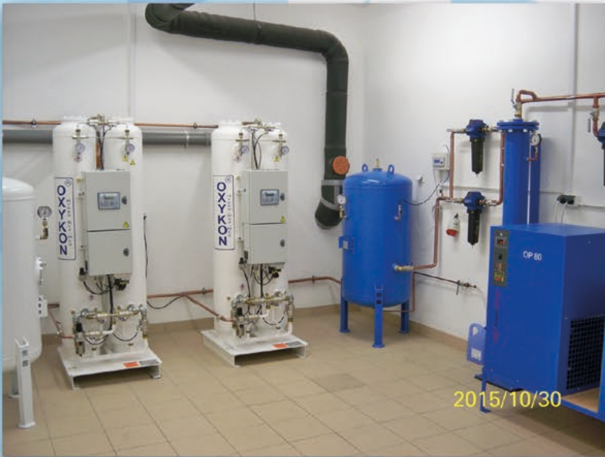
Oxygen concentrator system
