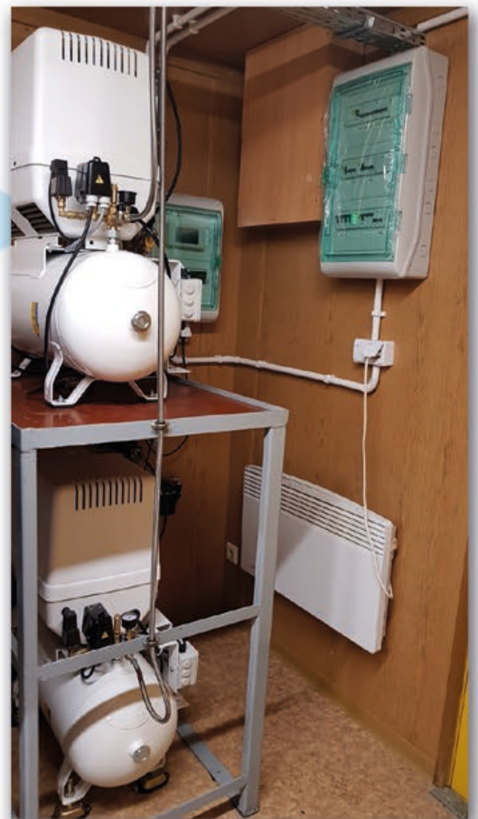
Medical air system in container
