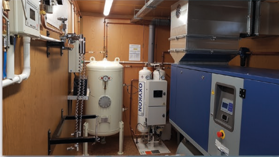
Oxygen concentrator system in container
