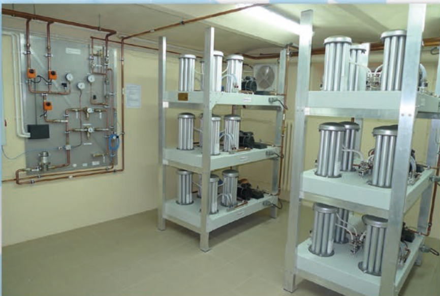
Oxygen modular concentrators system
