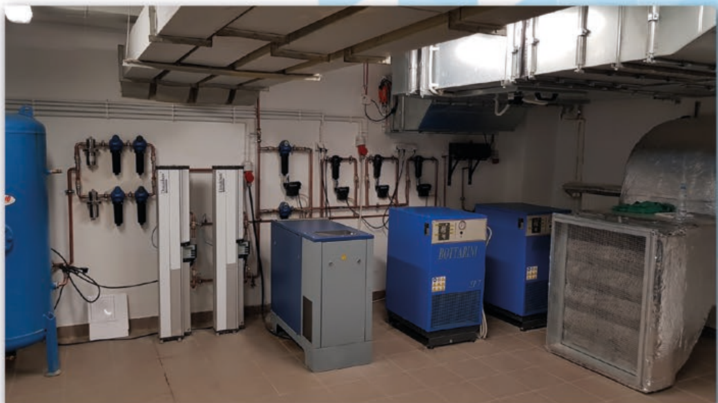
Medical air plant
