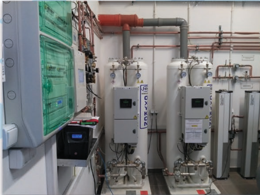
Oxygen concentrator system
