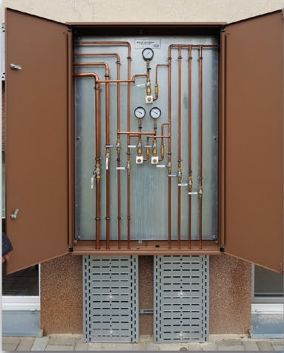
Maintenance and emergency node
