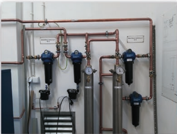
Compressed air treatment
