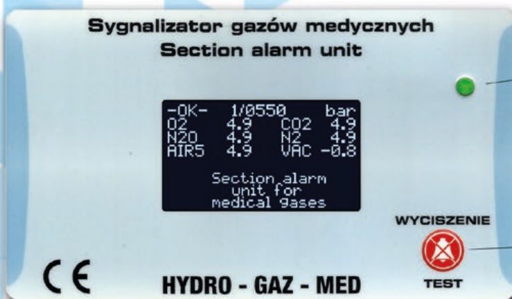
Section alarm unit
