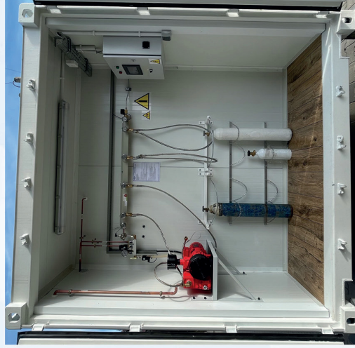
Cylinder filling station
