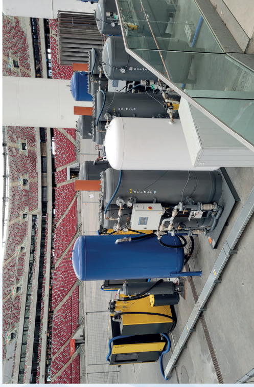
National Stadium in Warsaw - temporary COVID hospital
