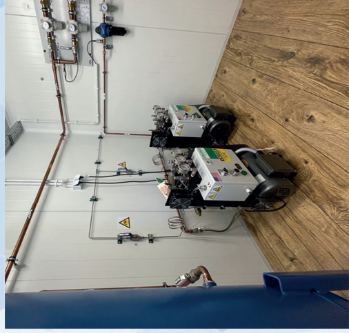
High pressure compressors
