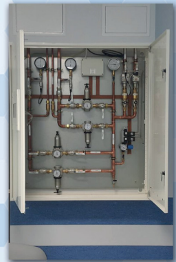
Oxygen control panel
