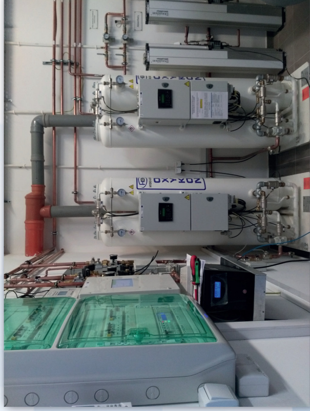
Oxygen concentrator system
