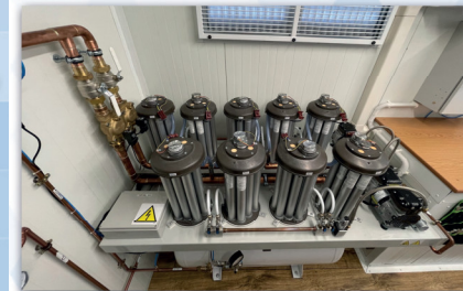
Oxygen modular concentrators system
