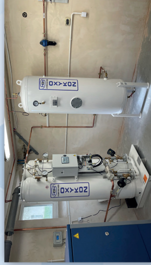
Oxygen concentrator system
