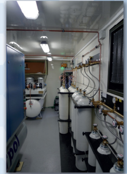
Oxygen concentrator and cylinder filling system in container
